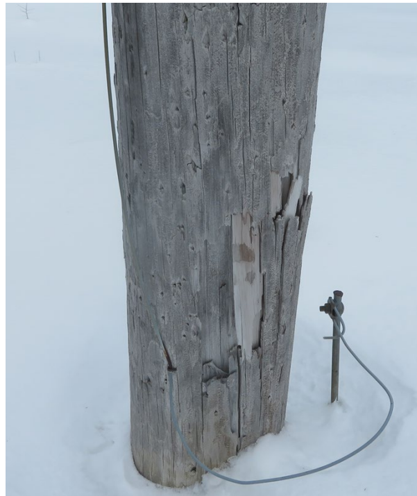
Figure C-3: Pole Deterioration
