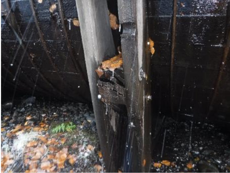
PHOTO 21 SPLIT SADDLE 69 DOWN FROM DAM ON LEFT SIDE
