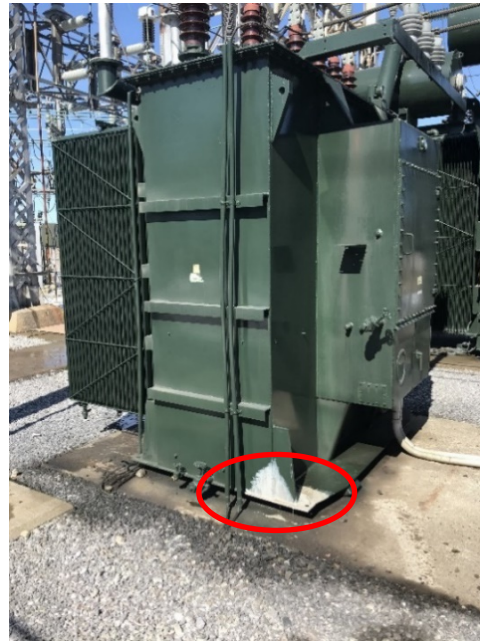
Figure 7: Leak Repairs on HUM-T2
