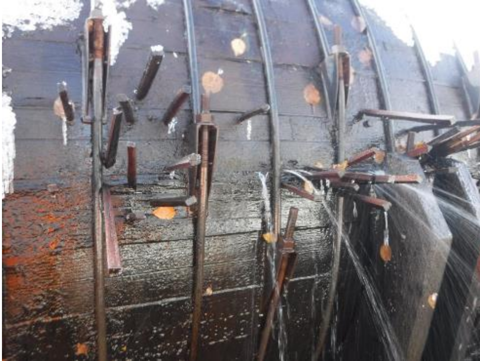
PHOTO 9 SEAM AND SPOT WEDGES UPSTREAM OF SURGE TANK
