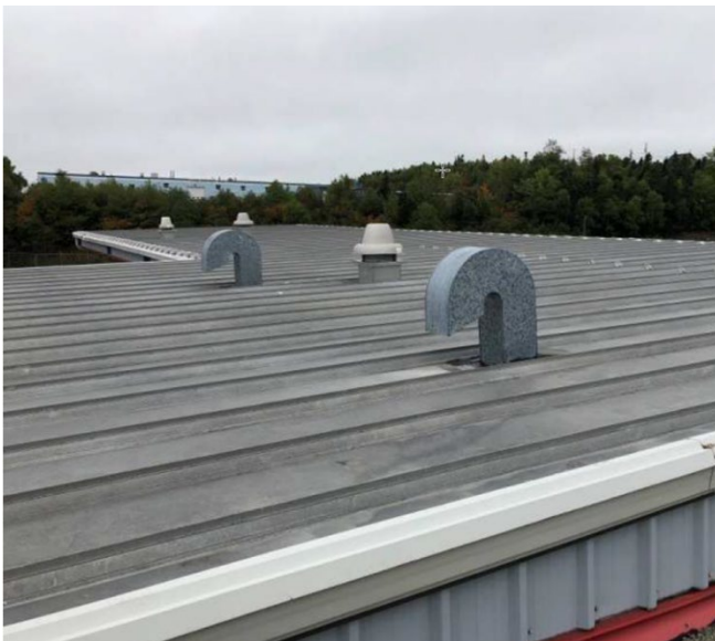
Figure 7: Warehouse/Maintenance Area Metal Roof
