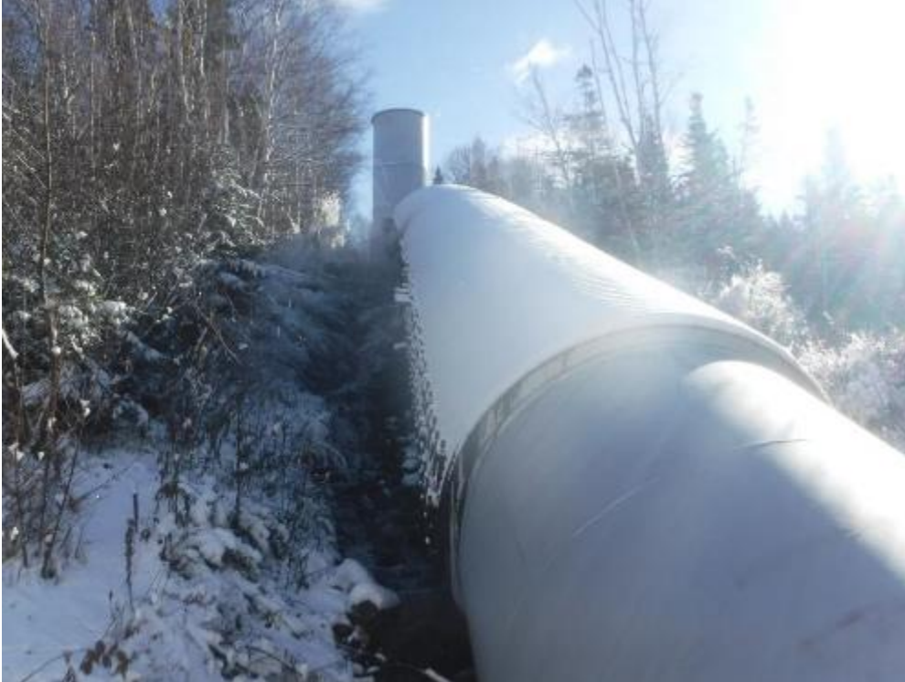
PHOTO 1 LOOKING UPSTREAM FROM POWERHOUSE ALONG RIGHT SIDE OF PENSTOCK
