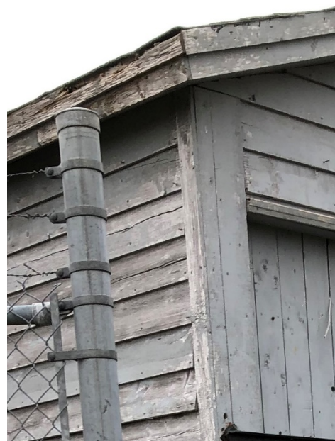
Figure 5: Deteriorated Eaves
