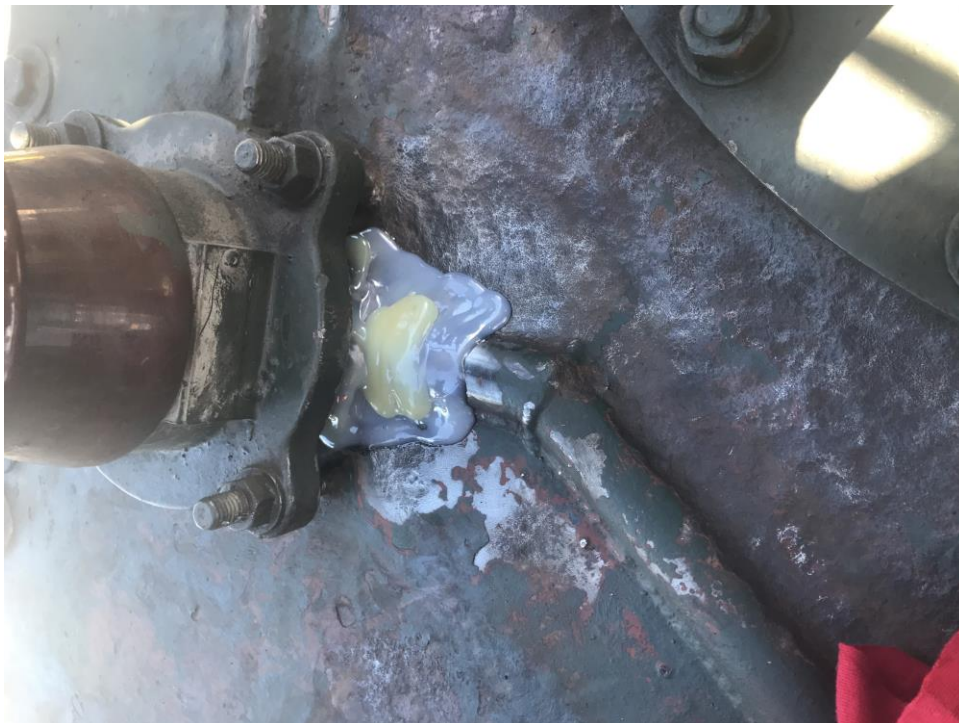
Hole in Transformer Tank Cover near Bushing – After Patch Application
