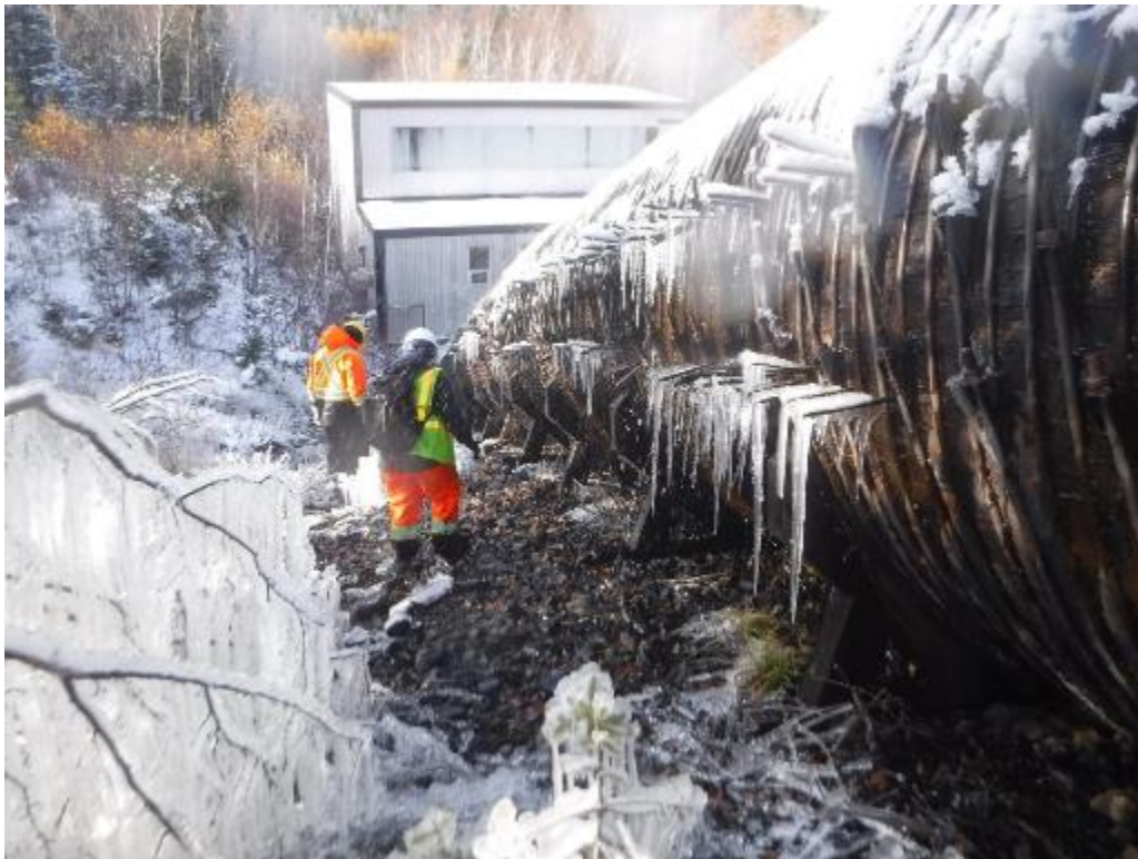
PHOTO 8 LOOKING DOWNSTREAM ALONG LEFT SIDE NEAR PH. NOTE WEDGES.
