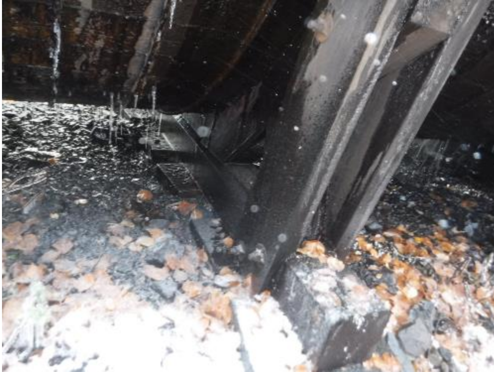
PHOTO 25 TYPICAL SADDLE FOUNDATION
