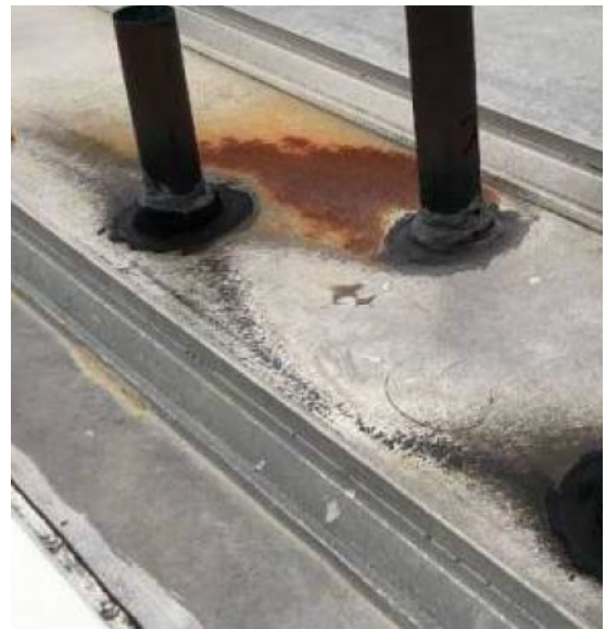
Figure 8: Deteriorated Sealants
