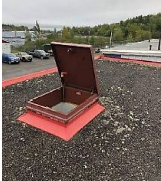
Figure 6: Existing Roof Hatch
