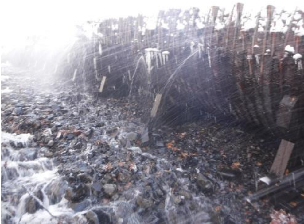
PHOTO 2 RIGHT SIDE OF PENSTOCK NEAR POWERHOUSE
