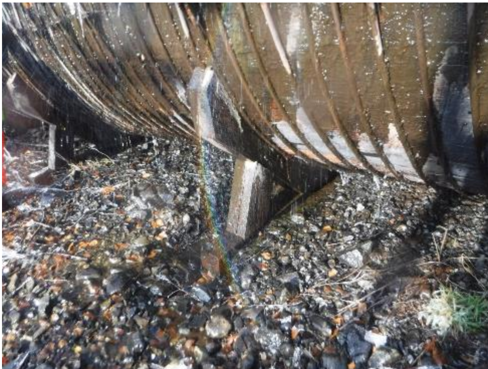
PHOTO 24 140 DEGREE SADDLE STYLE NEAR THE POWERHOUSE. TYPICAL BEDDING MATERIAL
