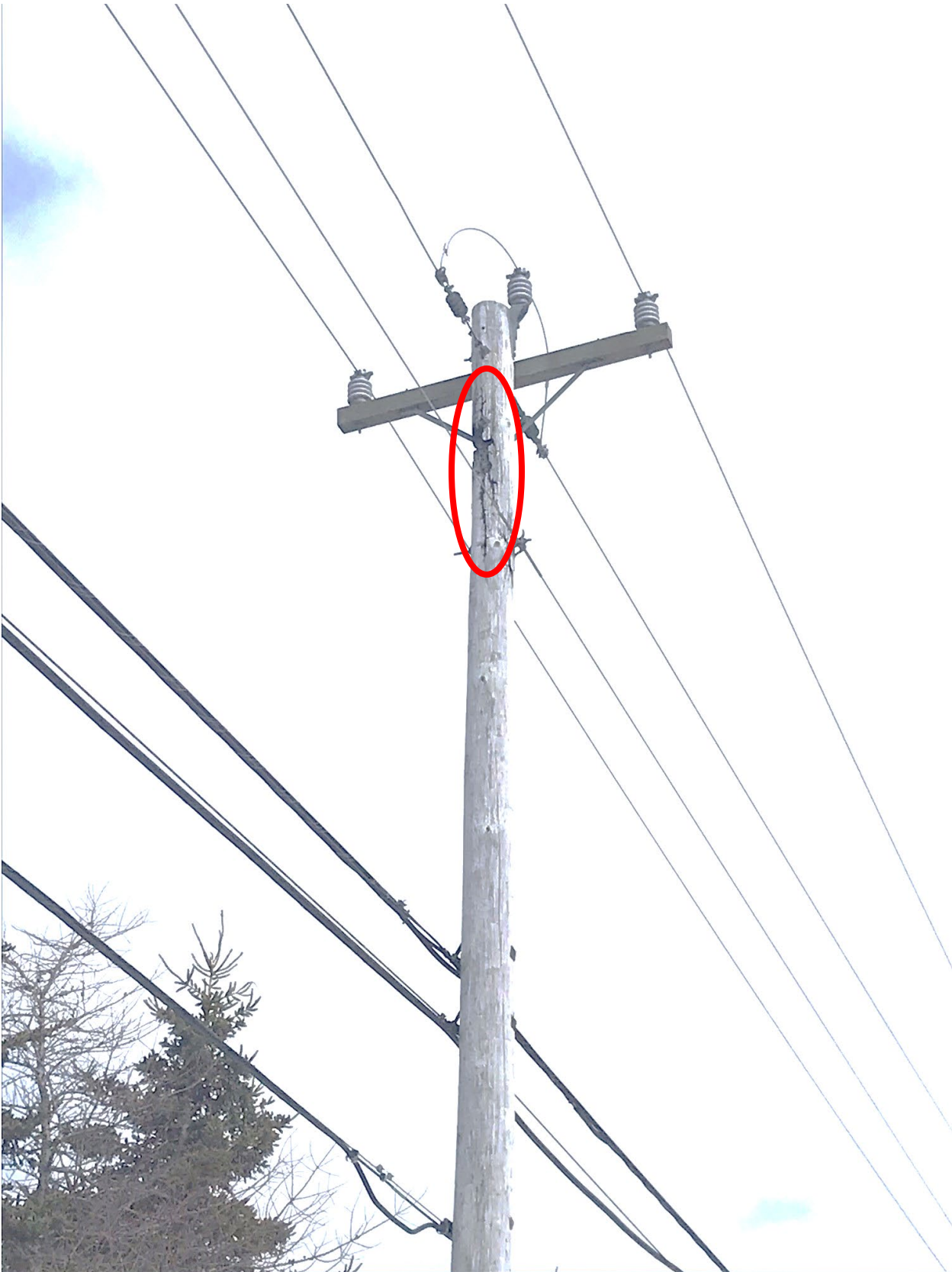
Figure B-4: Damaged Pole due to Insulator Flashover
