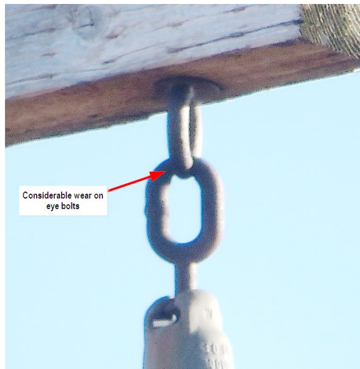
Figure C-12: Worn Ball Link Eye Bolt
