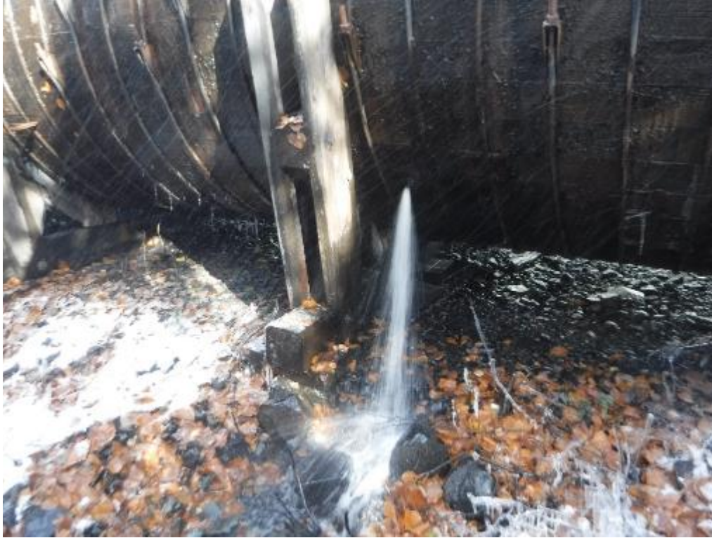
PHOTO 11 WATER JET ON LEFT ADJACENT SADDLE 34 NUMBERED FROM DAM
