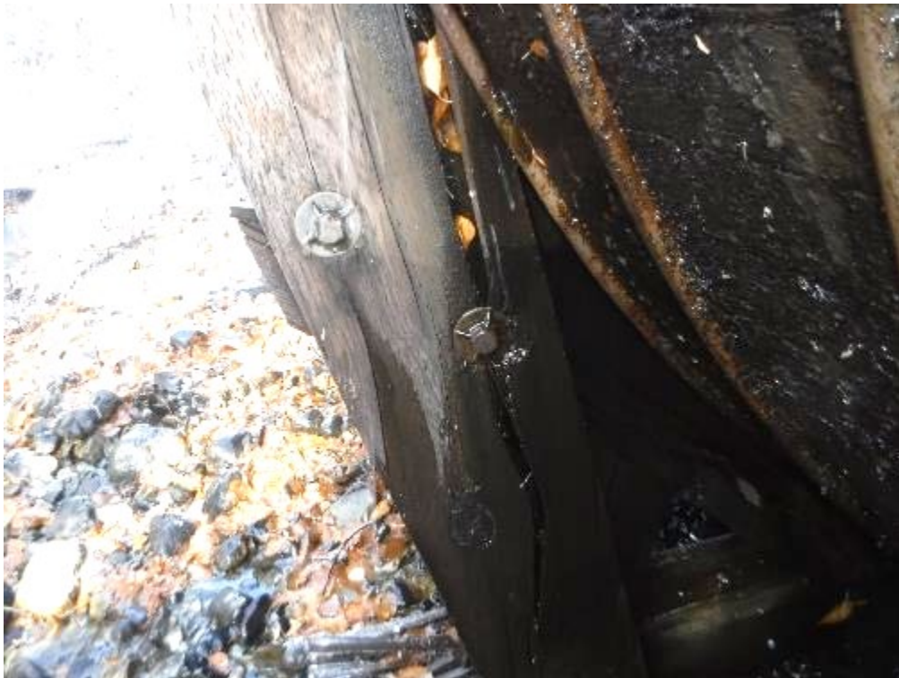
PHOTO 20 SPLIT VERTICAL 46 DOWN FROM DAM ON LEFT SIDE
