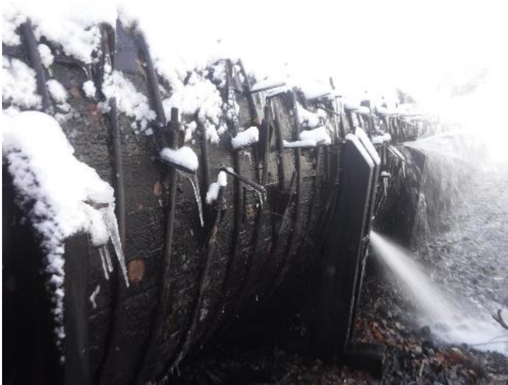
PHOTO 13 WATER JET ON RIGHT 30 METERS DOWNSTREAM OF SURGE TANK
